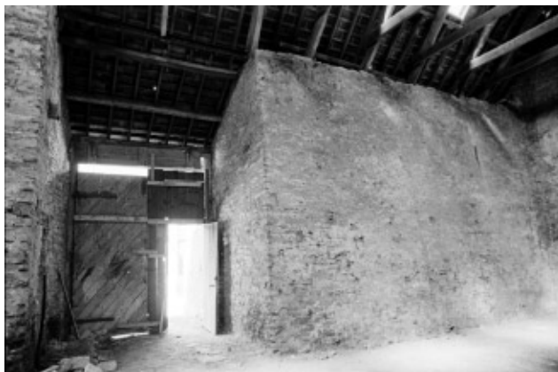
West door. The stub end of round beam projecting from the upper south west wall is thought to be the remains of the beam that supported a canvas sheet that could be swung like a Punkah to make extra draft for winnowing while threshing.
