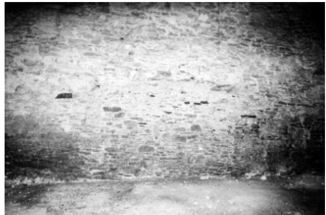
An unexplained belly into the south west wall. It does not appear to be a worn feature.
